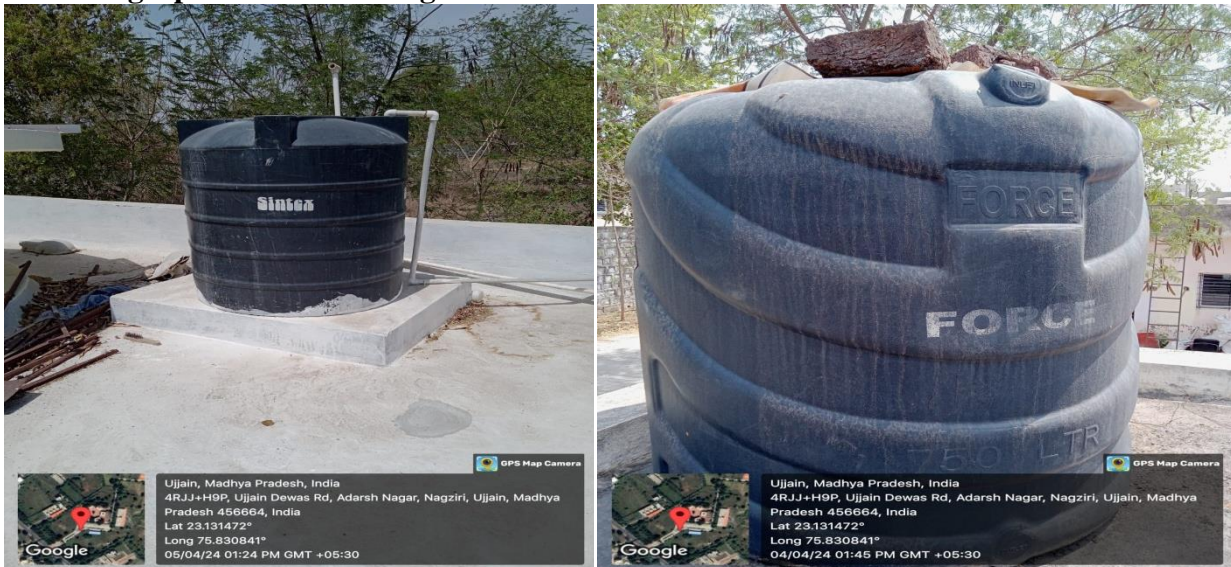
Water Storage Tank in the University Campus (Panchavati Pariser)
